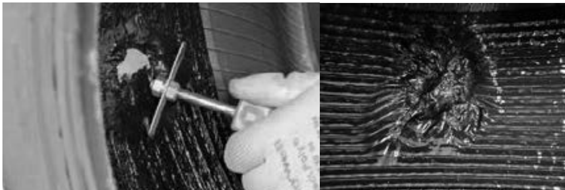
Figure 2 - Reposition sealant over repair area
